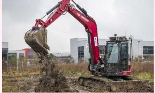
Figure 3: Autonomous Excavator in Construction Site
