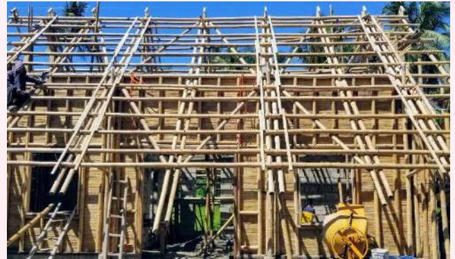
Fig 2: Bamboo structure eco construction
