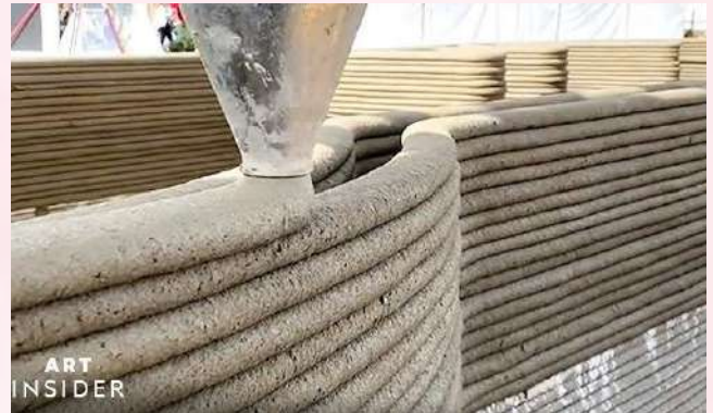
Figure 4: 3D Printed Building Structure
