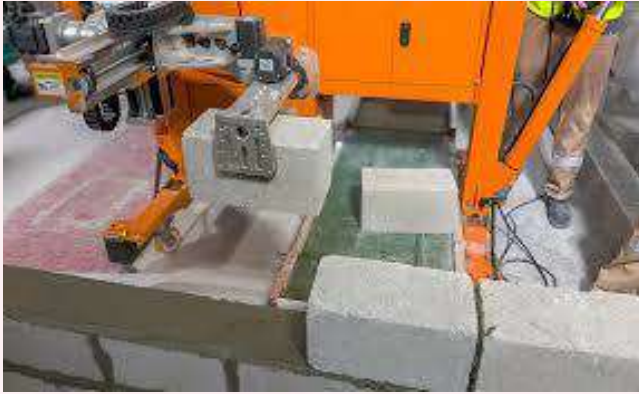
Figure 1: Robotic Bricklaying in Construction Engineering
