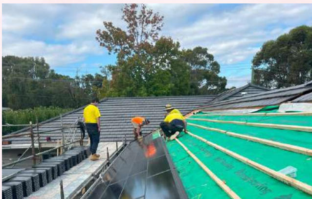
Fig 3: Solar panel roof installation
