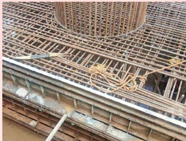
Reinforcement cages prepared for 2m diameter piles
