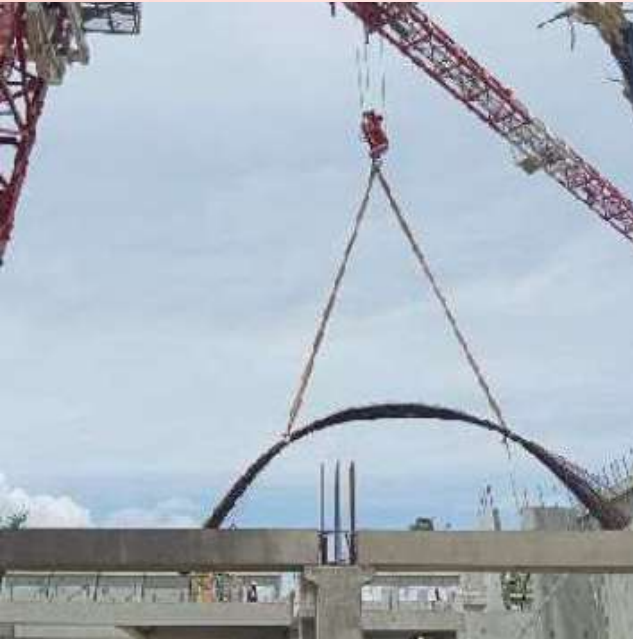
Precast panels being lifted and placed with the tower crane
