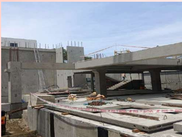
Slabs of precast commercial building
