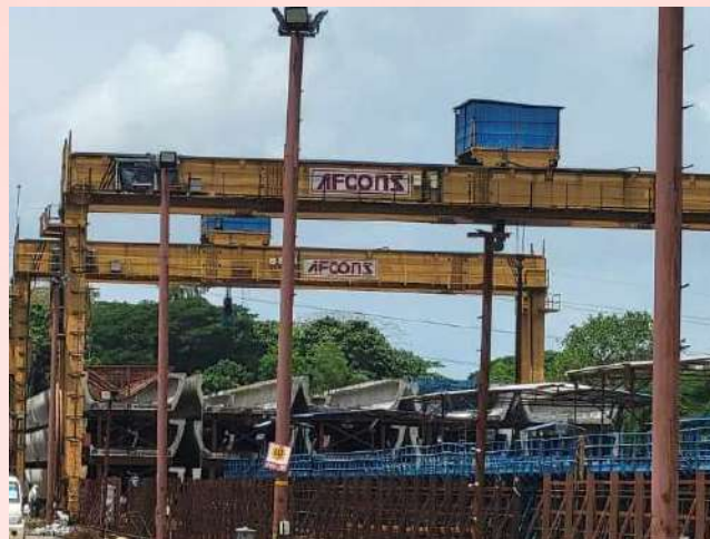
Casting bed for M55 grade U-girders at the precast yard
