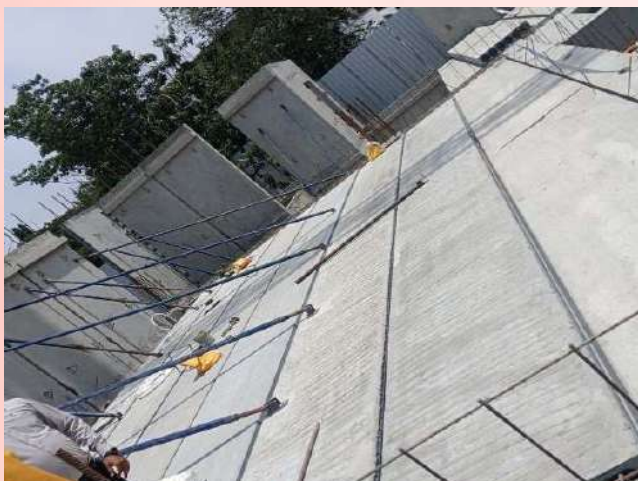
Slabs of precast commercial building
