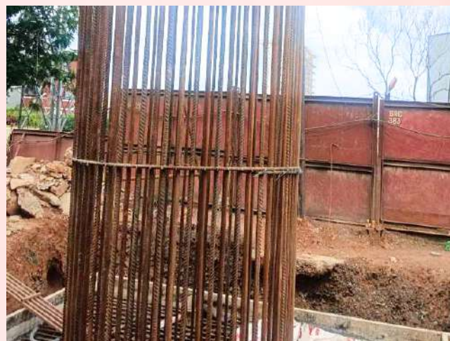
Reinforcement cages prepared for 2m diameter piles
