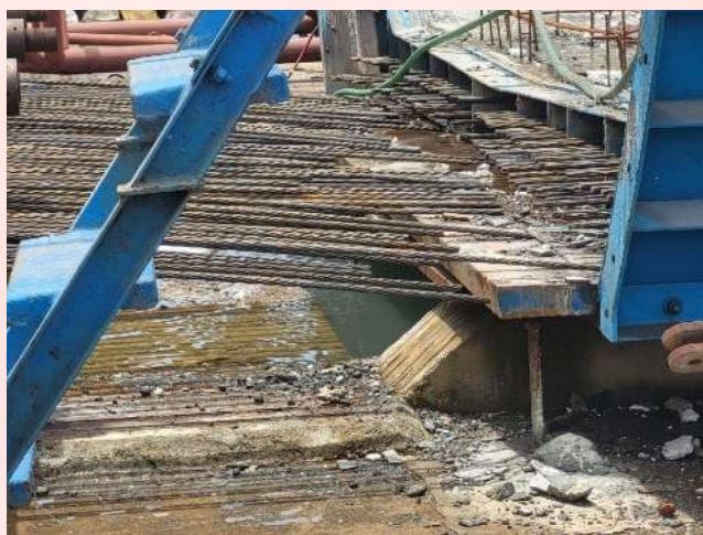
Casting bed for M55 grade U-girders at the precast yard
